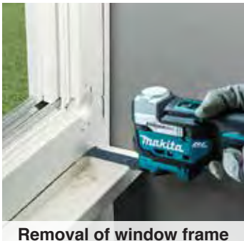
Removal of window frame
